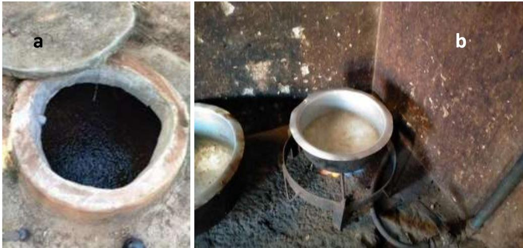
**Figure 10.** (a) Biogas digester. (b) Biogas stove.
